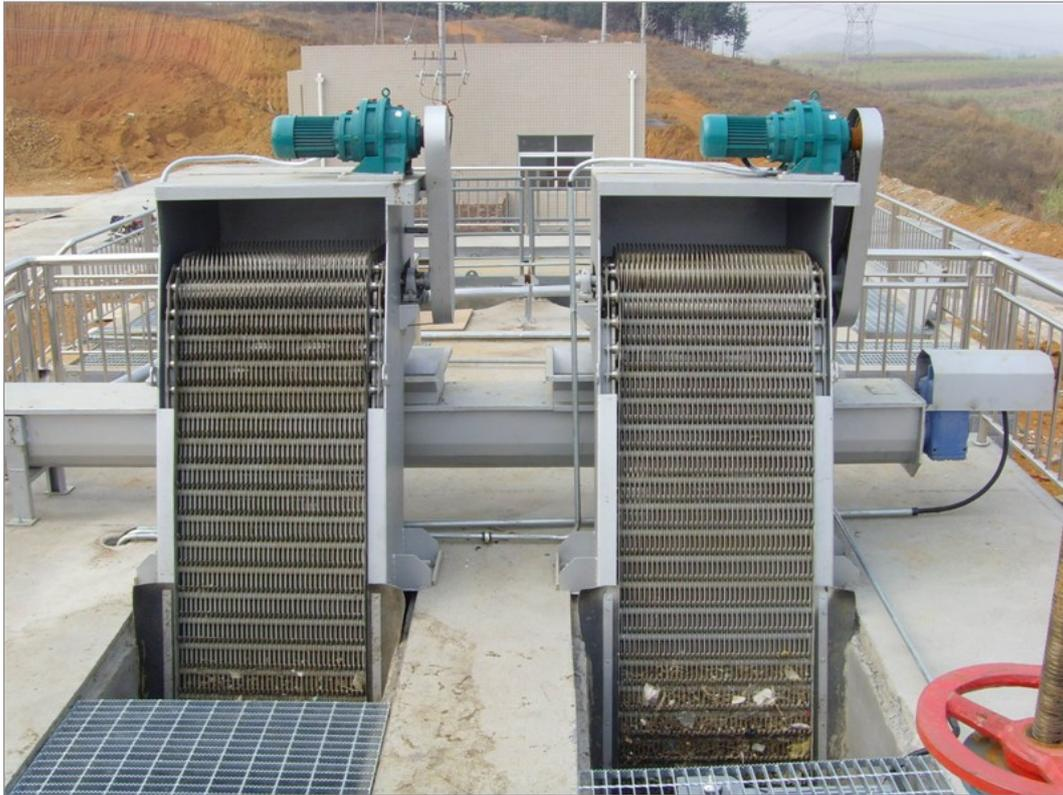
QY series automatic mechanical traveling bar screen is a filter for preliminary treatment, designed to remove debris and other inorganic material from the wastewater to protect downstream treatment process.
